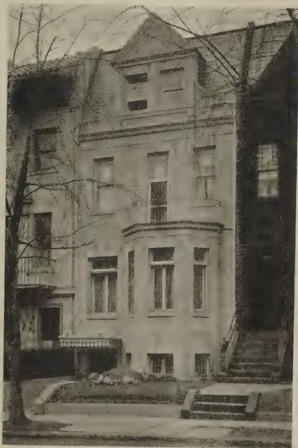
OLD BRICK HOUSE OVERCOATED WITH EXPOSED AGGREGATE STUCCO, WASHINGTON, D. C. THIS IS THE FIRST INSTANCE IN WHICH THE MOLDINGS WERE BUILT OF STUCCO OF THIS TYPE
